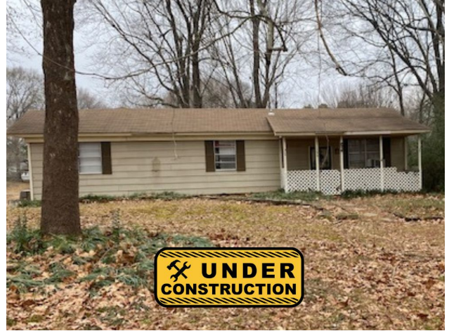
This home is under renovation and scheduled to be completed on: 05/02/21
