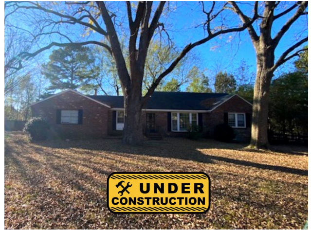
This home is under renovation and scheduled to be completed on: 02/15/21
